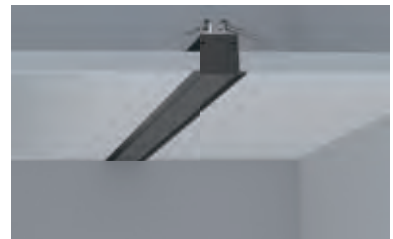
固定灯体，将灯体放入槽内 Fix the lamp body, put the lamp body into the slot
