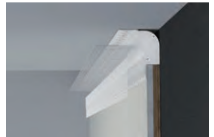
贴防裂网 Stick anti crack net
