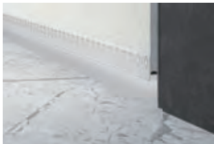
贴防裂网 Stick anti crack net
