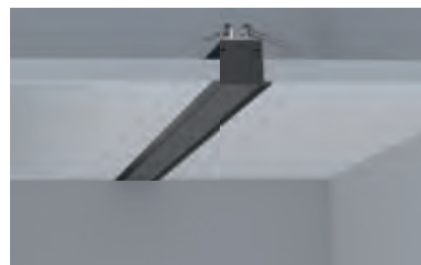
固定灯体，将灯体放入槽内 Fix the lamp body, put the lamp body into the slot
