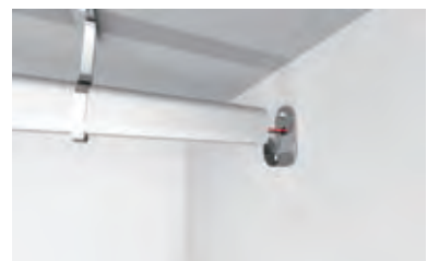
固定灯体，连接驱动电源 Fixed the light on wall ,connect driver and switch on
