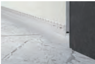
螺丝固定铝材 Fix the aluminum profile with screws
